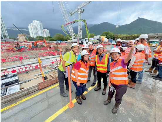
The delegation visited the works site of MTRCL Tung Chung Line Extension.
